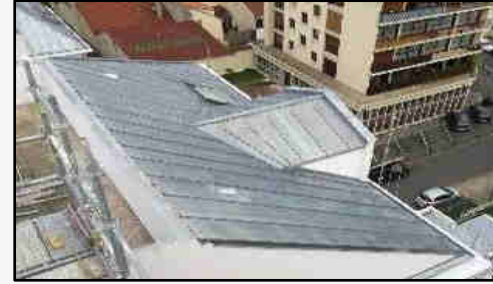
Rue Pierre Curie Alforville (94) - LOGIAL
